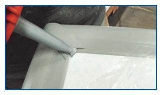
Apply a bead of caulk to the intersection of tabs and miters; smooth with your finger.
