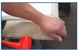
Immediately mount gasket on panel by spreading rigid legs of edging at one end and push onto panel. Using a wood block and hammer or mallet, tap into place progressively. Repeat block and hammer or mallet procedure several times the entire length of edge to assure snug installation.
