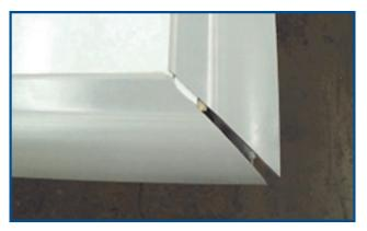
Cut replacement edge extrusion to fit (measure carefully). A small (1/8") expansion gap is required at each end.
