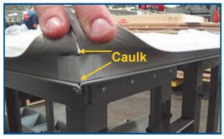
Install corner angle at all corners of edge. If the angle is wider than the panel thickness, cut to fit. Apply a 3/16" bead of adhesive on the inside of both sides of corner. Add a small bead of caulk to seal the top and bottom of the corner angle.
