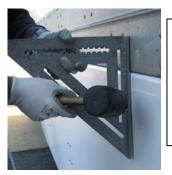
Align the skirt to the base-rail with a straight edge. A rubber or plastic non-marring mallet may be used to adjust the skirt's position only when a single bolt is snugged. Adjusting a skirt with a mallet that has been fully clamped down may cause damage to the skirt or cross-member clamps.
